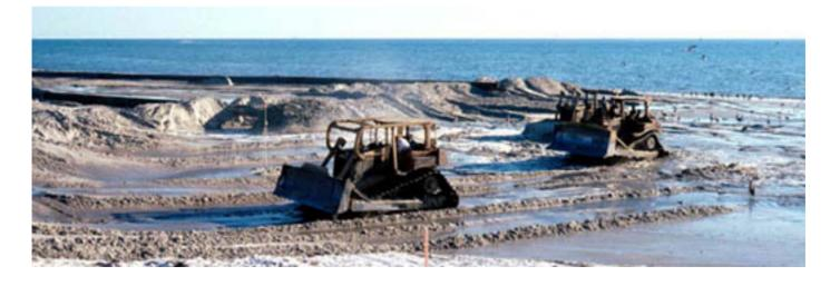
The replacement sand is usually dredged up offshore and transported to the beach
