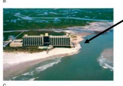
Notice the small concrete seawall built to "protect" the hotel from the inlet
